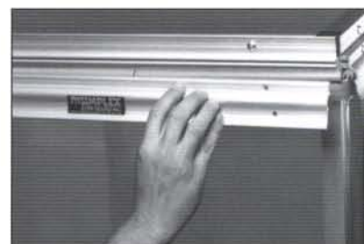
3. Attach front plate with machine screws provided. Your installation is complete.
